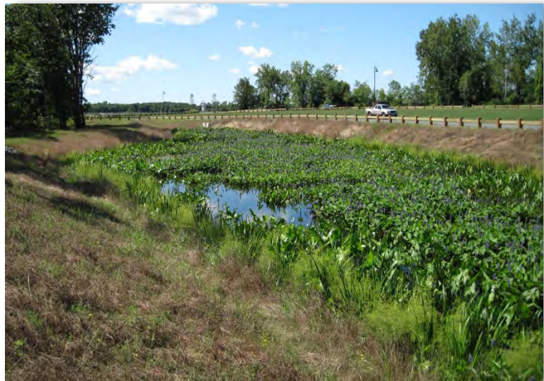
Example of a Water Quality Detention Basin
