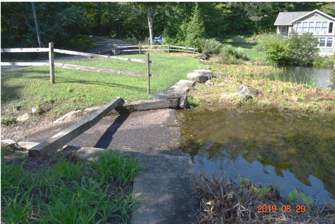
Photo 12b – The right side training wall for the left side spillway.
