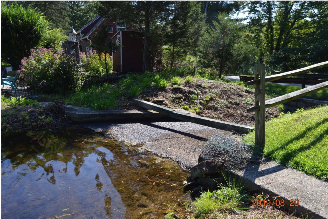
Photo 9c – Looking downstream at the left side spillway and its environs.
