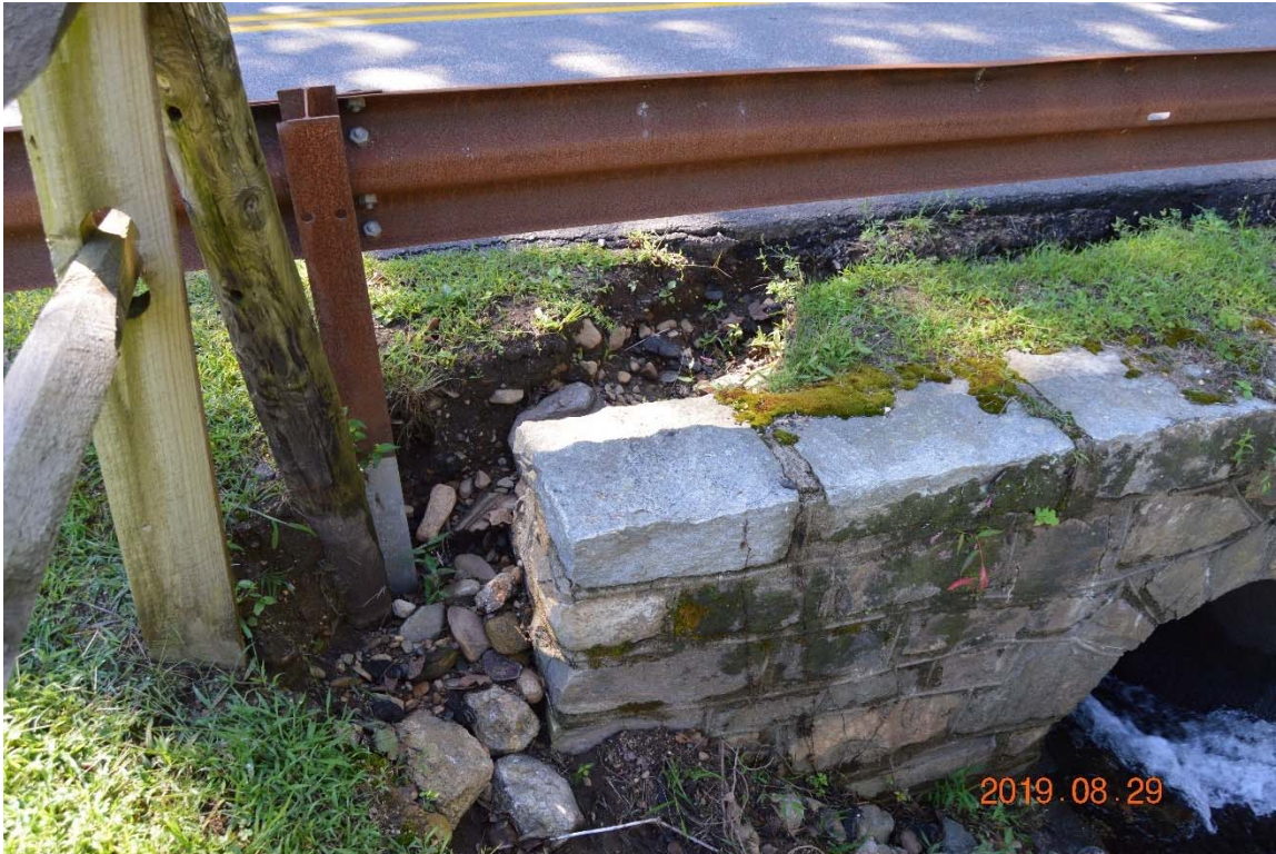
Photo 21c – An area of washed out soil, caused by runoff from Haywardville Road, running around the right side discharge culvert endwall at the time of inspection. This area was subsequently repaired (see below).
