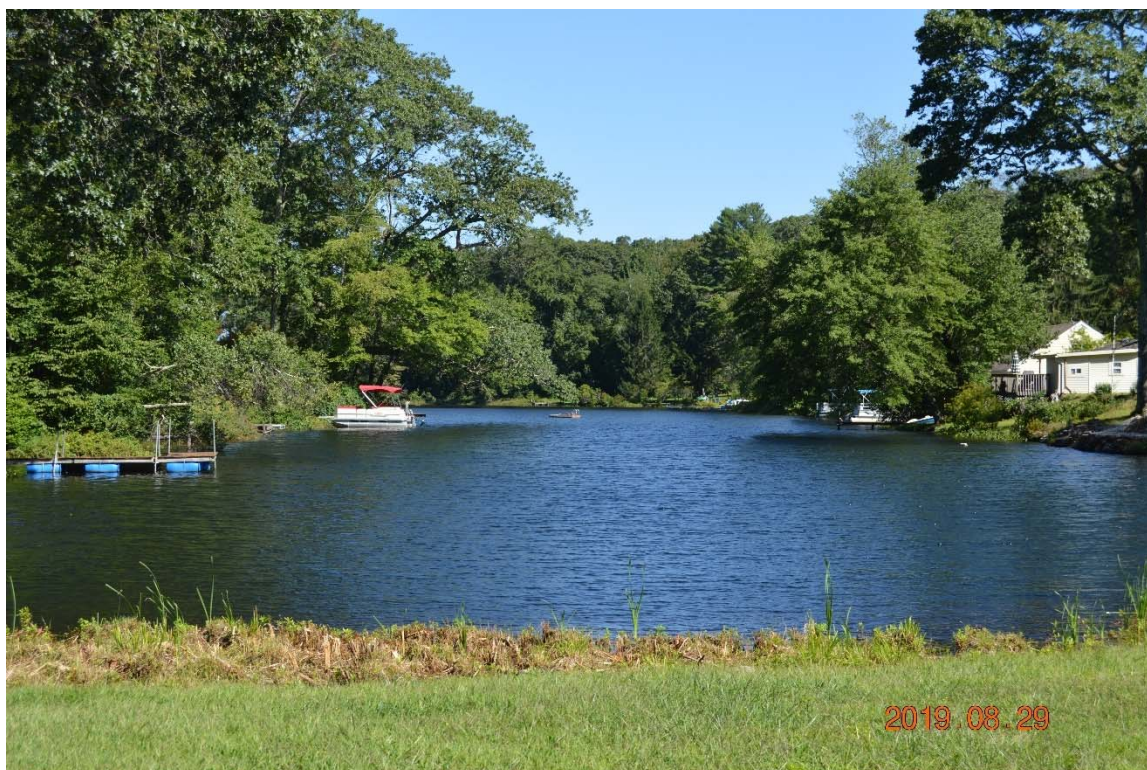
Photo 20b – Looking upstream at Lake Hayward from the center of the embankment crest.
