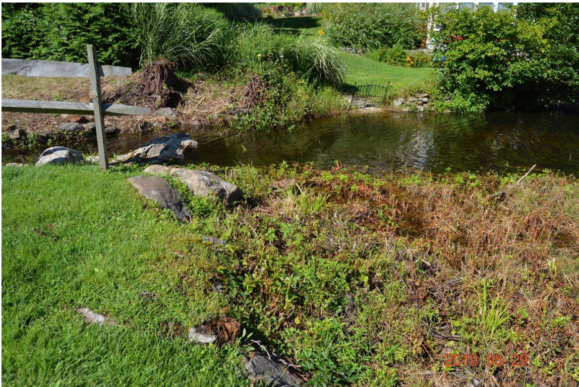
Photo 9d – The right side spillway as seen from the upstream side (partially obscured by flow).
