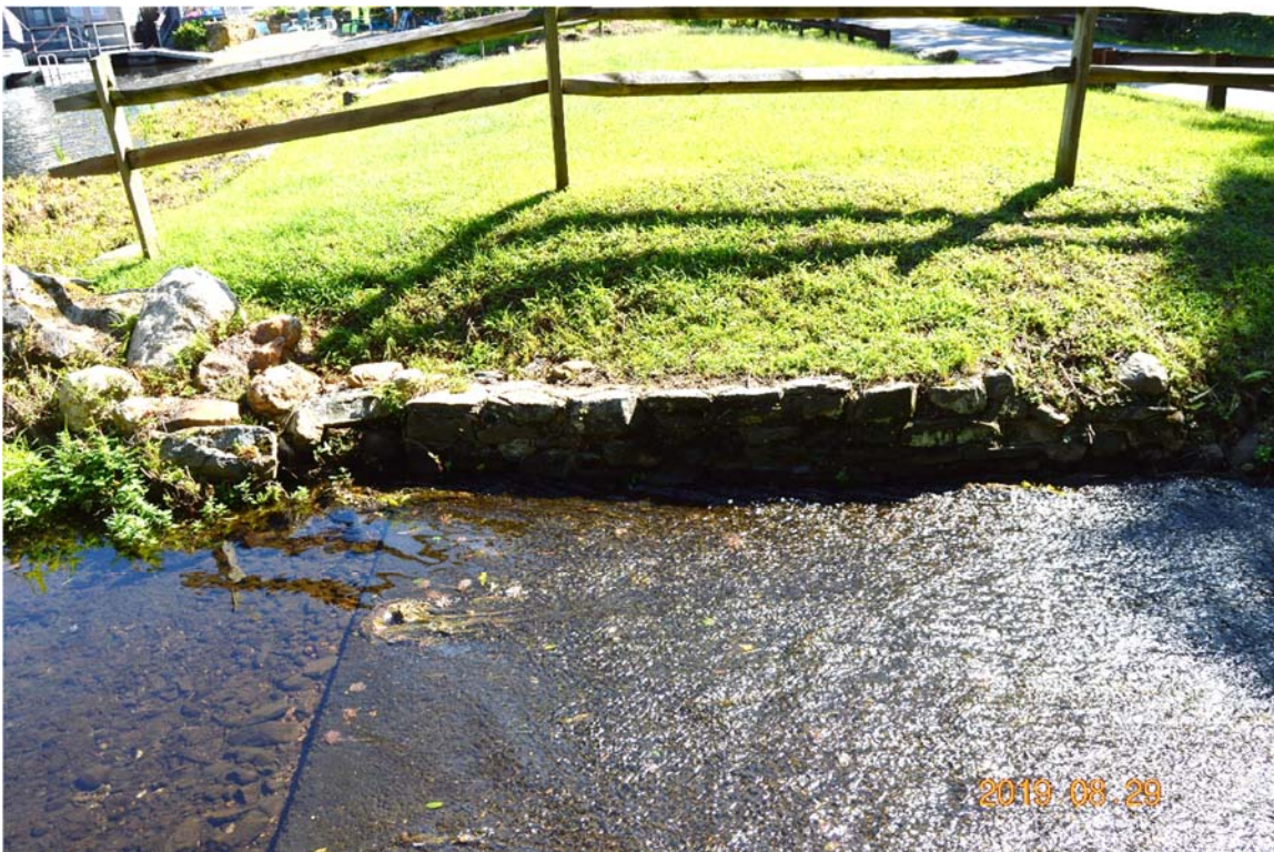
Photo 13b – The right side spillway weir.
