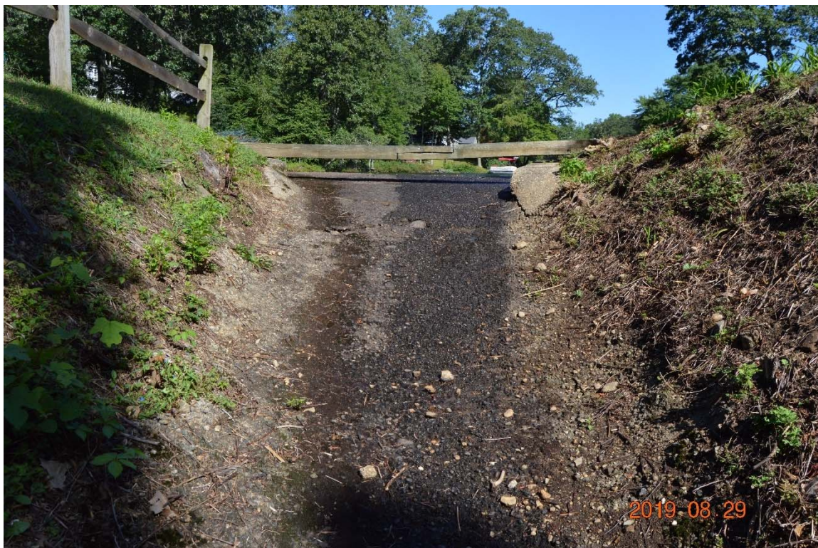
Photo 10b – The left side spillway, as seen from its discharge channel.
