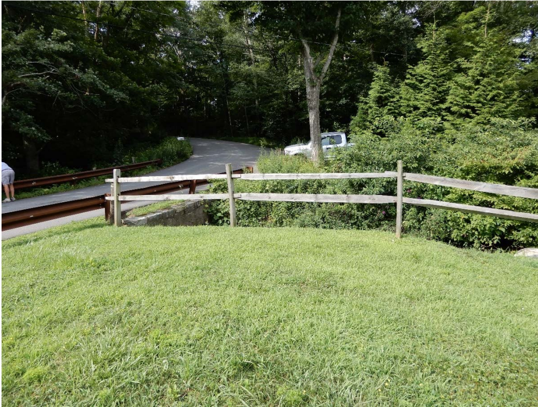
Photo 5b – The right end of the embankment crest.
