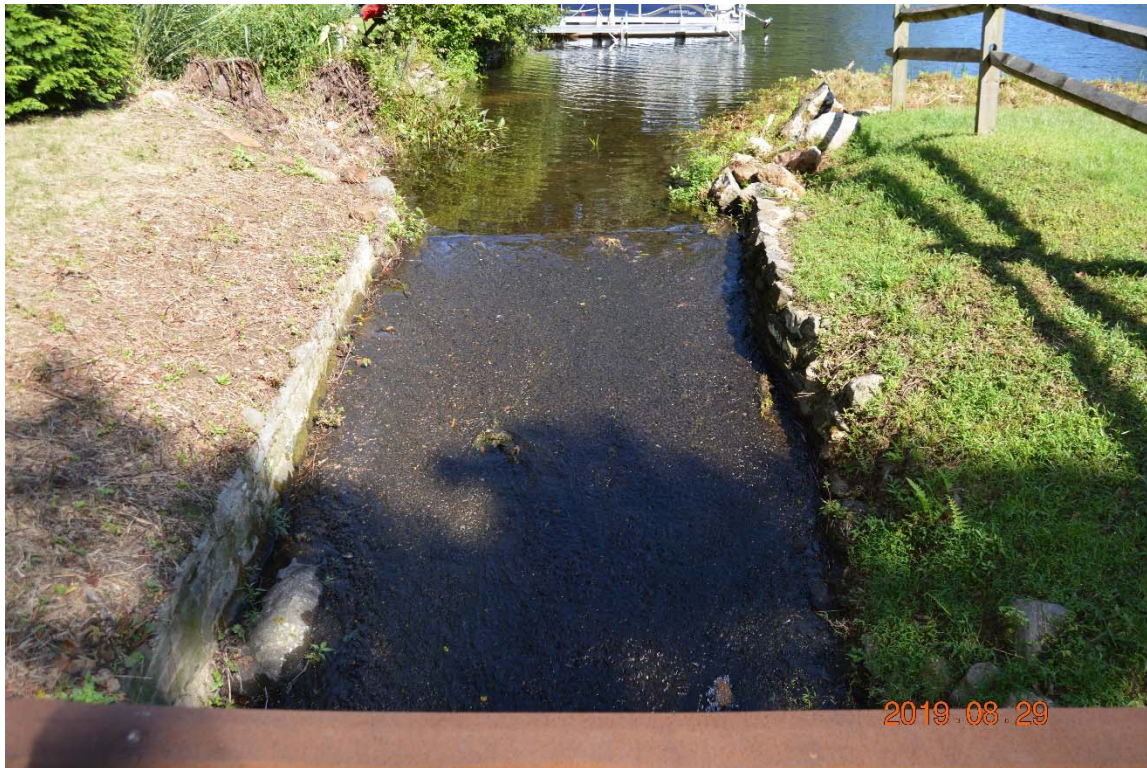
Photo 10c – The right side spillway as seen from the downstream side.
