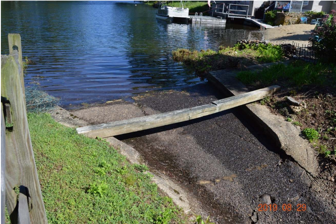
Photo 13a – The left side spillway weir.
