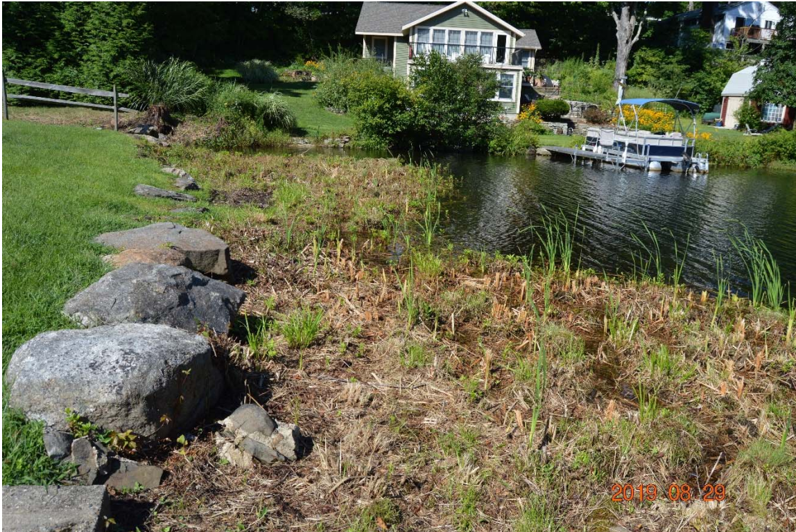
Photo 4d – An overview of the upstream embankment as seen from the left side.
