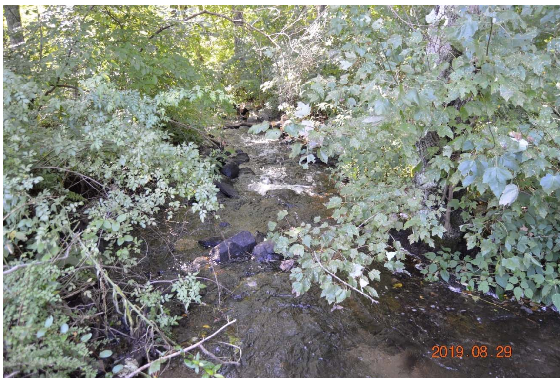
Photo 15e – A close up view of the right side discharge channel.
